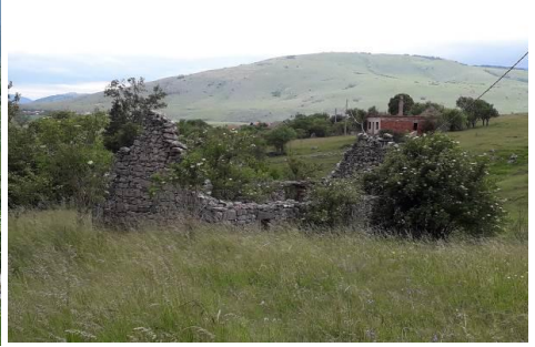
(D) Black elders sprouted from the collapsed buildings
